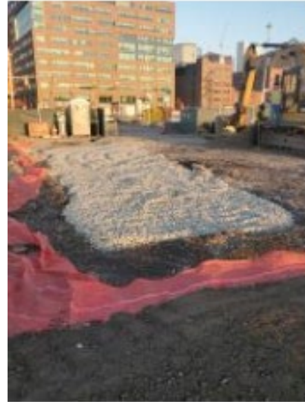
Backfill of decontamination TSCA Area after excavation
