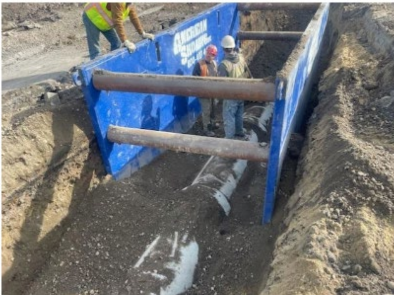
Drainage installation in trench box
