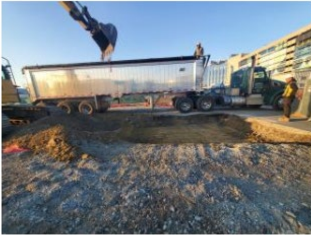
Excavation in TSCA Area
