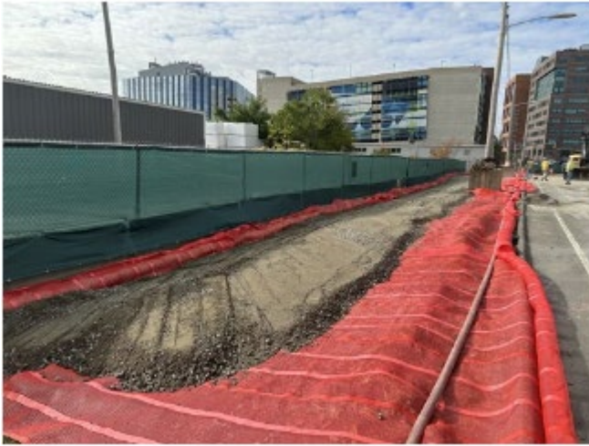
Southside liner and fill in TSCA area
