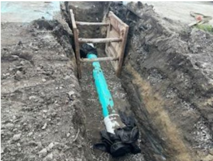
Drainage line in D to E Connector
