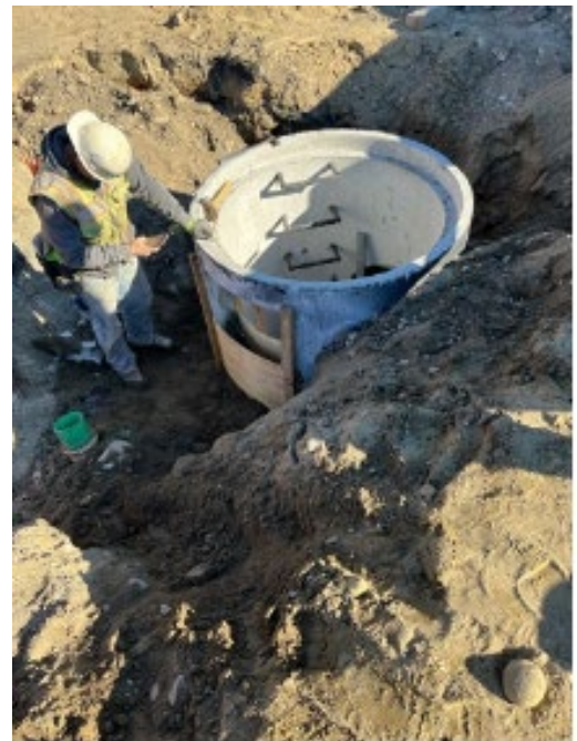
Manhole in D to E Street connector
