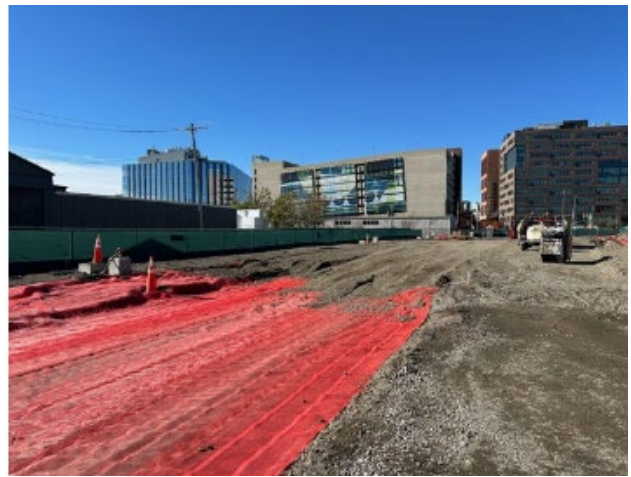
Backfill over linear in TSCA Area
