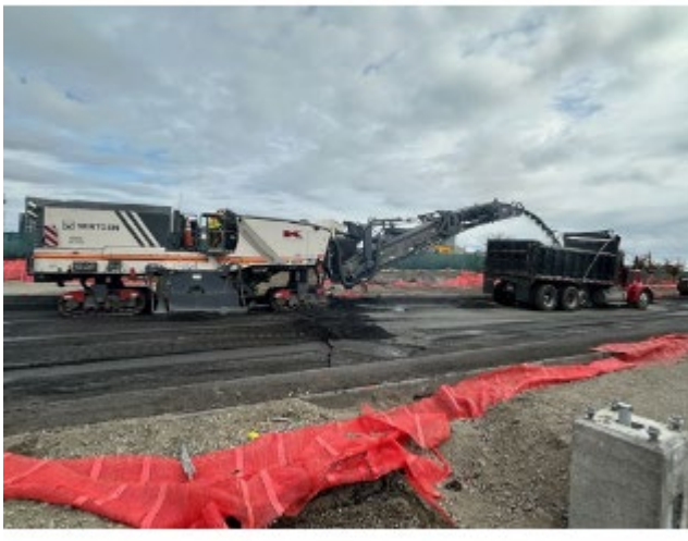
Asphalt milling in TSCA
