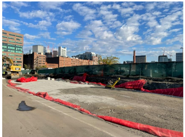
Backfill with linear in TSCA area
