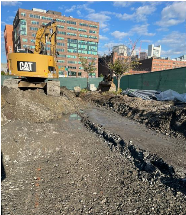
Moist soil in TSCA Area excavation
