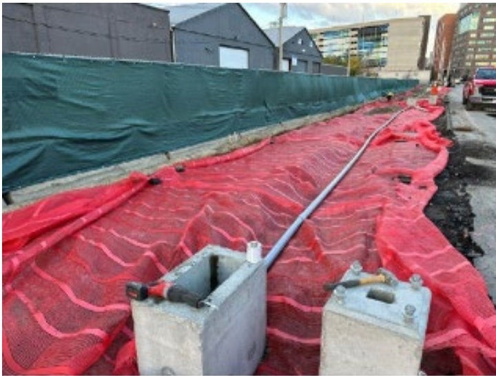
Light pole base above marker layer in TSCA Area
