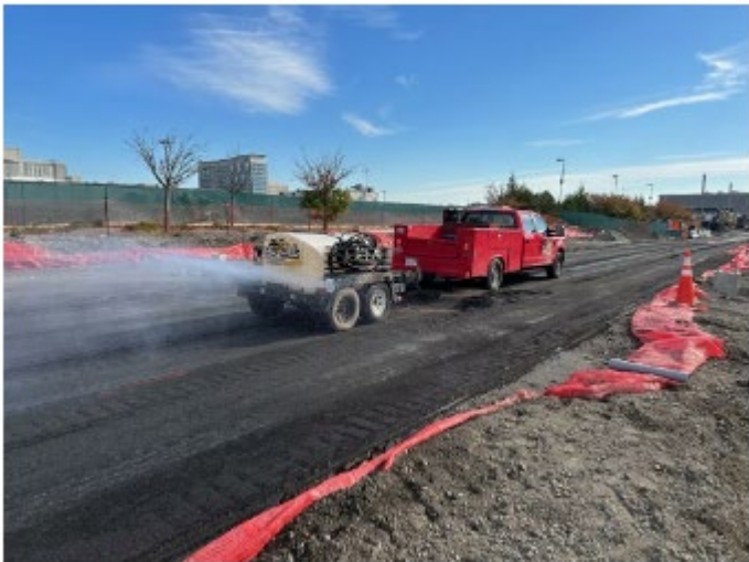
Water misting during milling
