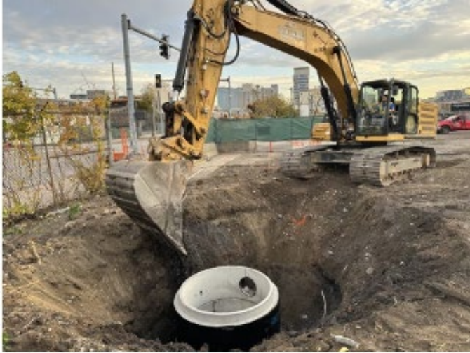
Catch basin in C to D Connector
