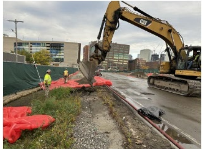
Placement of marker and linear on South side of TSCA area
