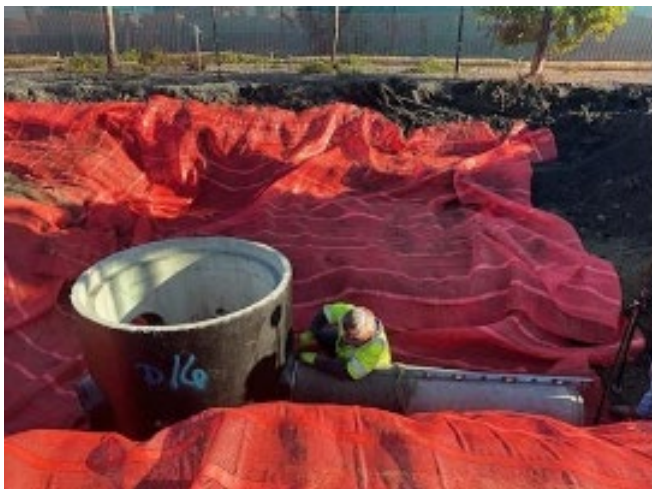
Catch basin in roadway in TSCA area over marking layer
