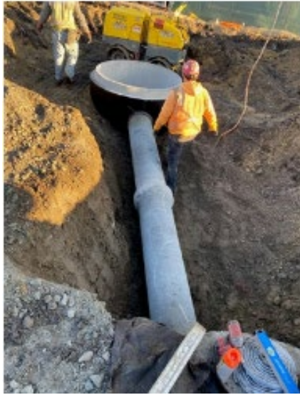
Continued placement of drainage structures between Bullock and D Street
