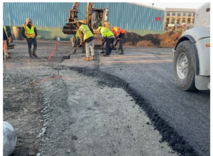
Asphalt paving in C to D Connector
