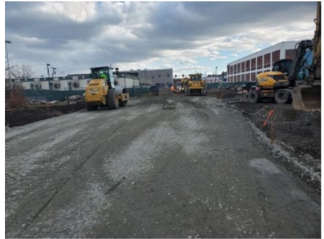
Final grading before paving
