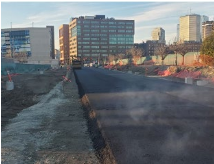
Asphalt paving in TSCA Area
