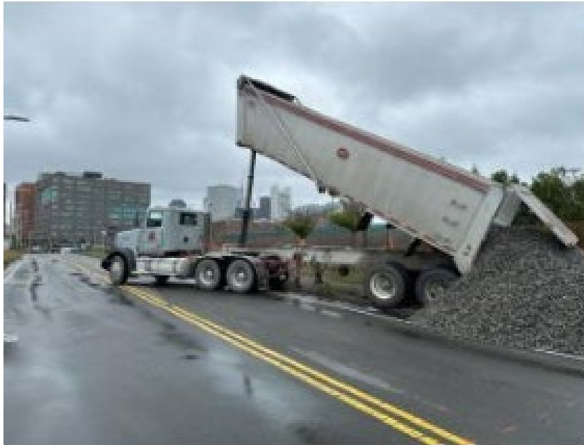
Trailer Dump Load of ¾" stone
