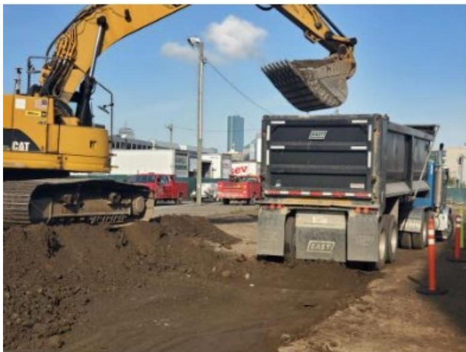
Excavation and Loading in D to E Connector
