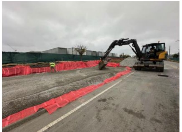
Excavation in TSCA Area that has been Backfilled
