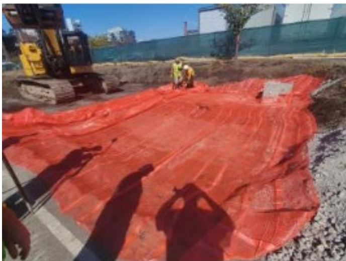
Marking Linear Before Backfilling in TSCA Excavation
